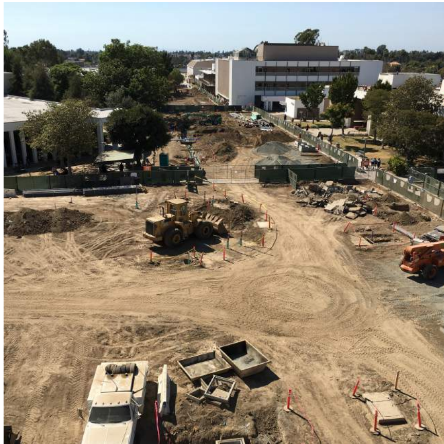
Phase 5 Construction Zone
