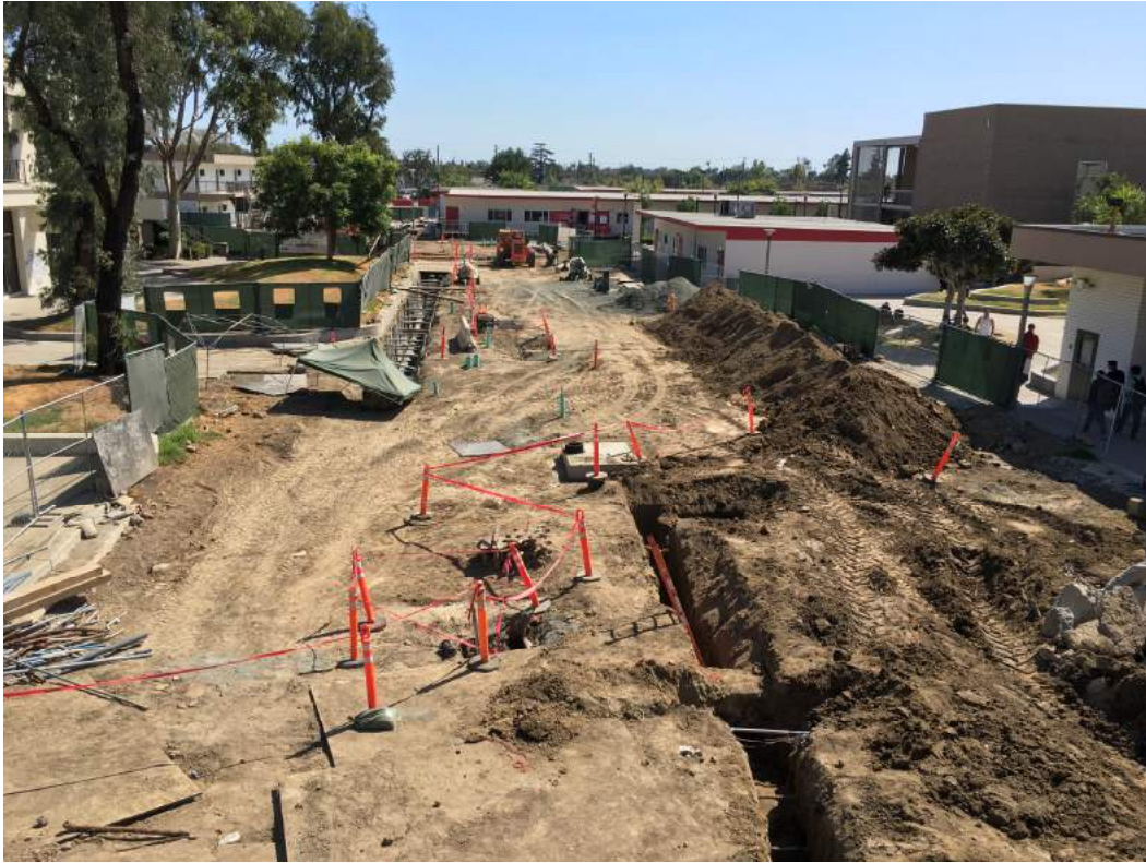
Phase 4 Construction Zone
