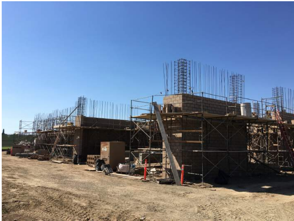
Central Plant Construction Zone
