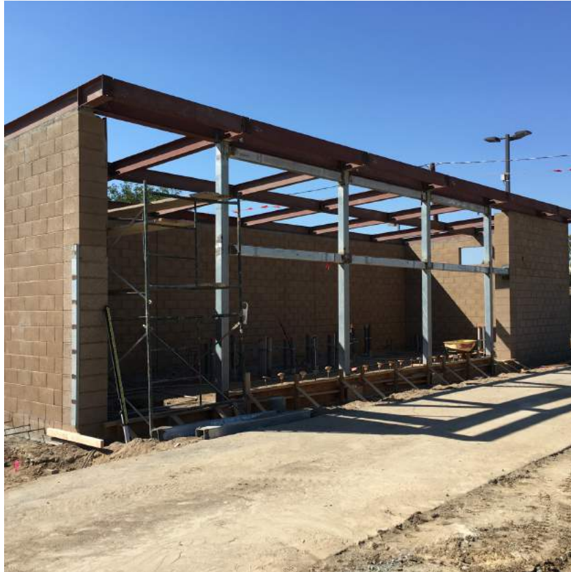
Electrical Building Construction Zone
