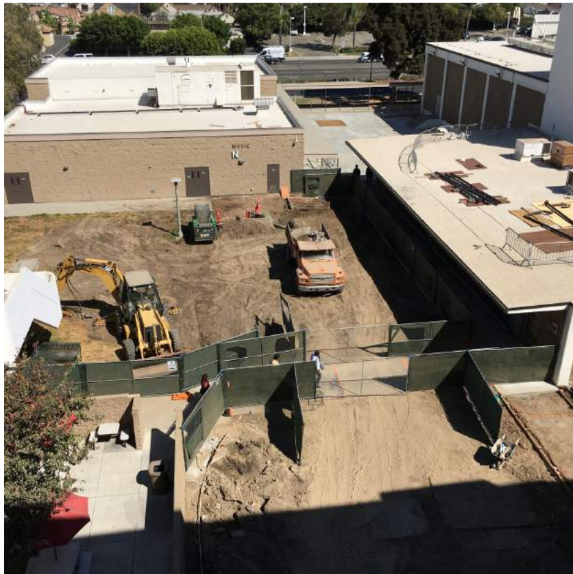
Phase 3 Construction Zone
